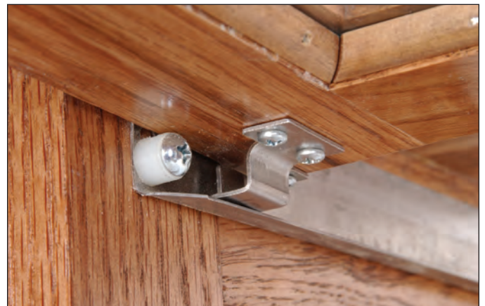
Left capture bracket shown mounted with the door open.
